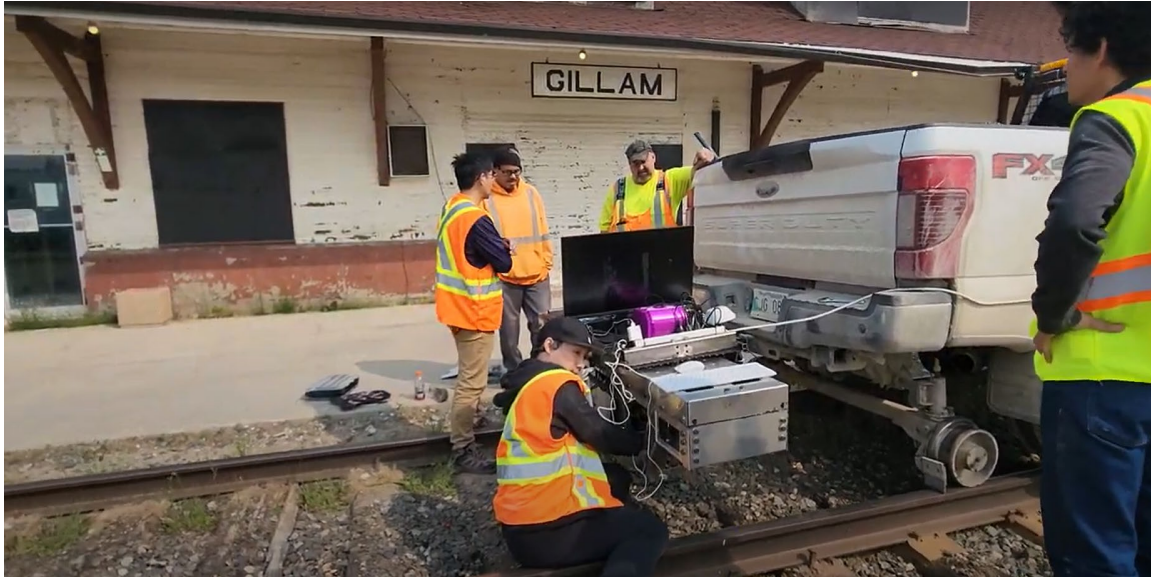
Figure 1: Inspection Truck installation at Gillam
